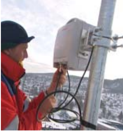
Figure 8 Installing MINI-LINK.
