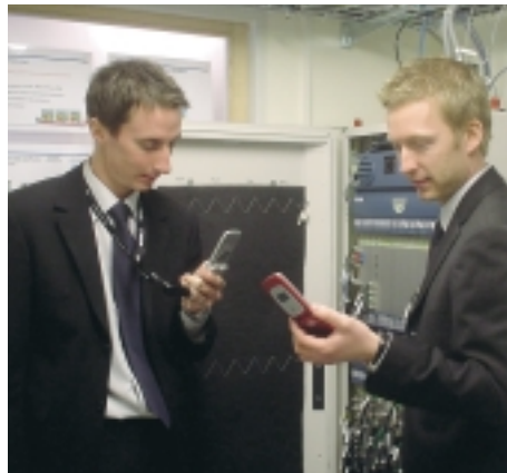
Figure 3 Interoperability of mobile terminals and network equipment from different vendors is crucial for handover between WCDMA and GSM. Ericsson network equipment, in commercial operation in Japan since 2002 (here represented by the Indoor Macro RBS 3202), has been publicly shown (at 3GSM World Congress in Cannes, February 18-21) to interoperate in WCDMA with all major mobile terminal vendors—here represented by two Sony Ericsson Z1010 terminals.
