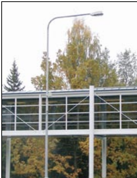
Base station integrated into lightpole
