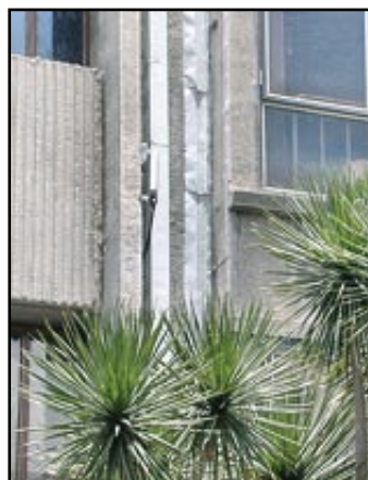
Base station blended into building facade
