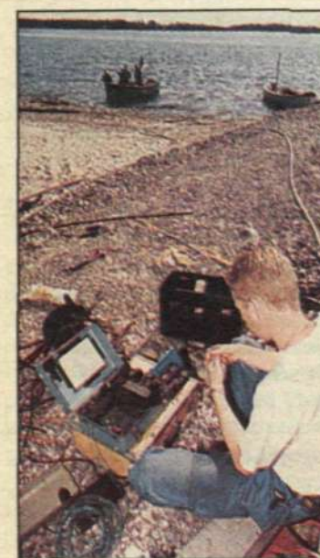
Anders Holmberg at the controls of the measuring equipment used to check that the fiber cable is in impeccable condition.
