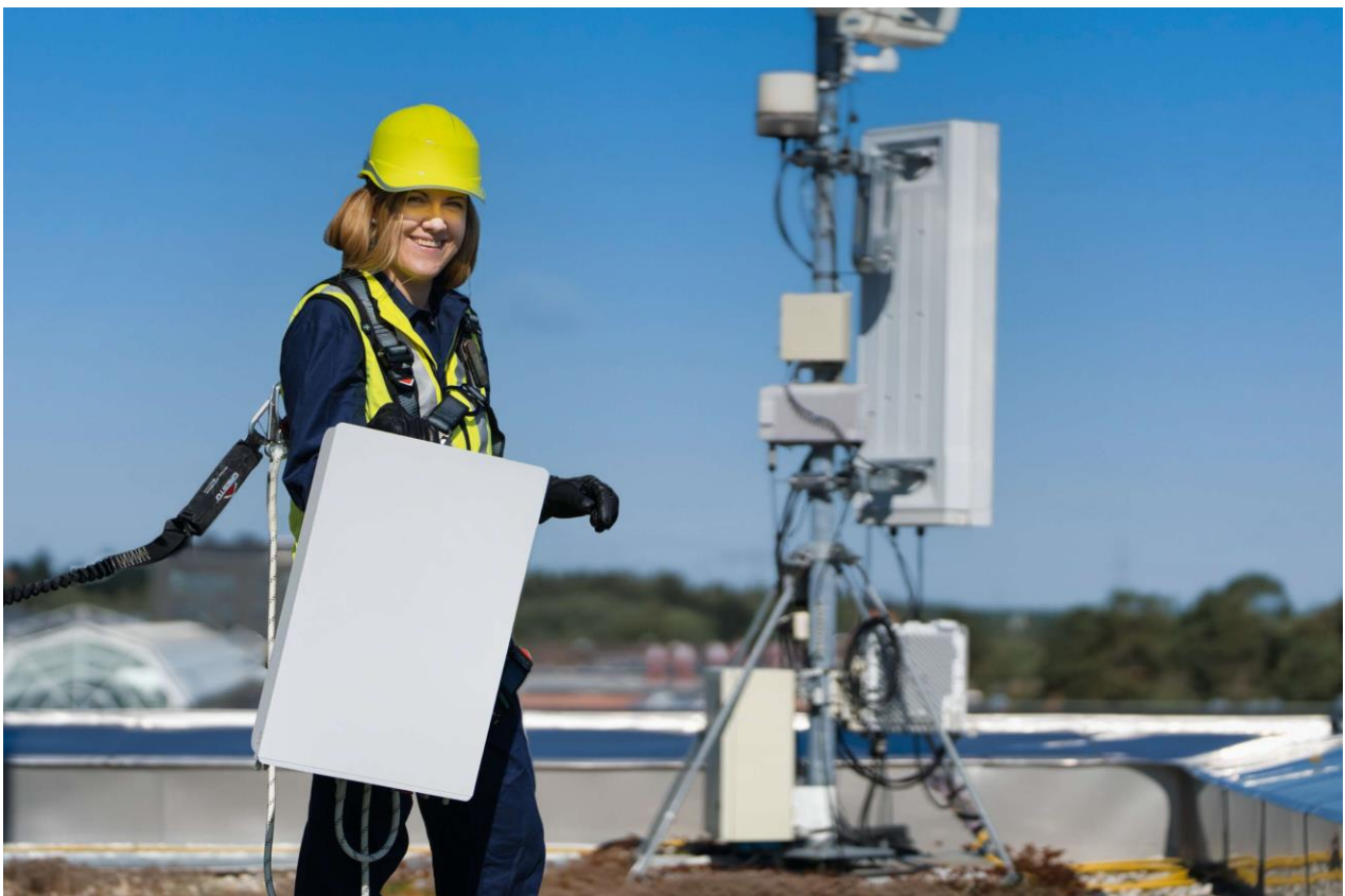
Ericsson Air 3268 radio rollout on a rooftop.
