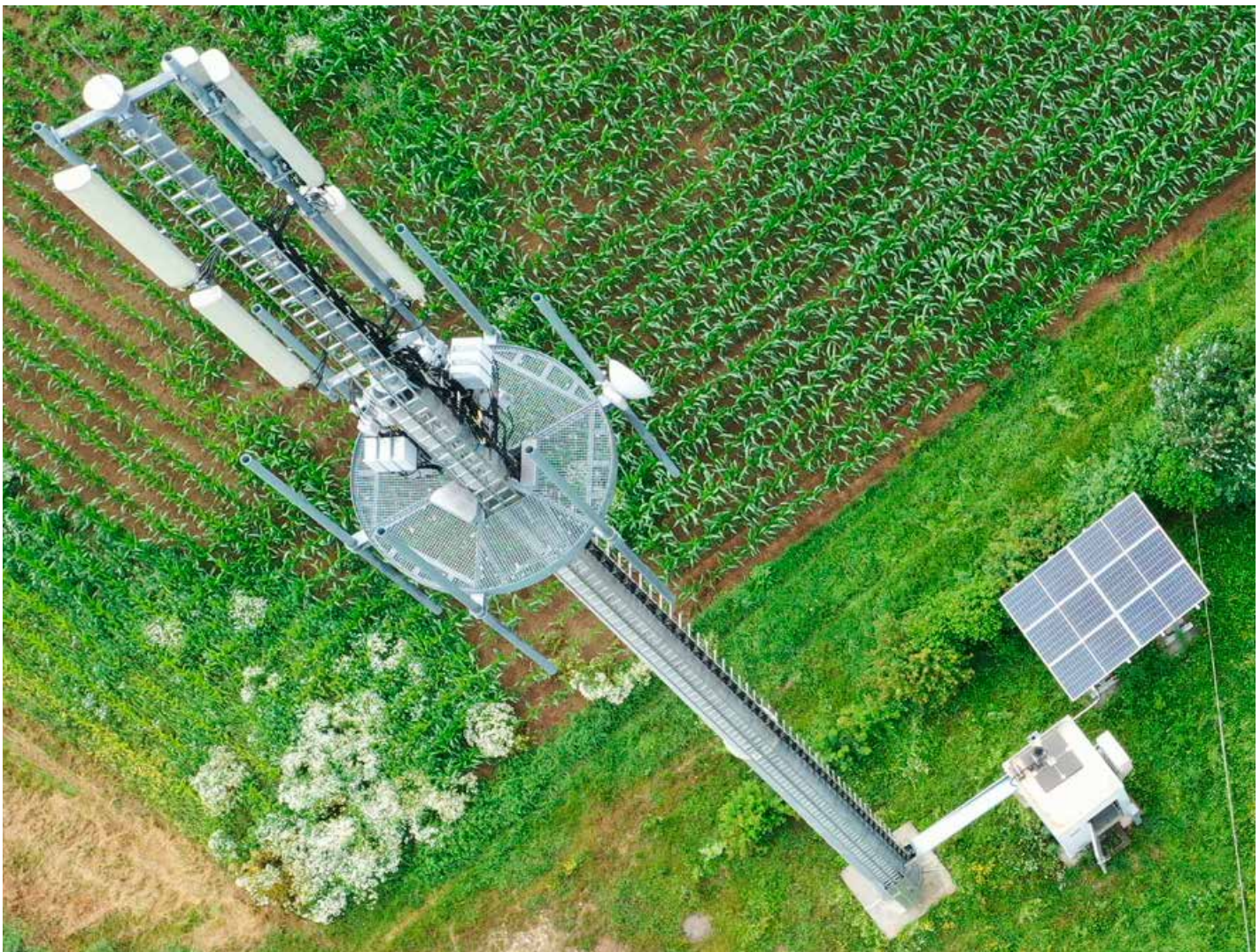
Ericsson and Deutsche Telekom have partnered to bring solar panels to a RAN network site. Image source: DFMG Deutsche Funkturm GmbH.
