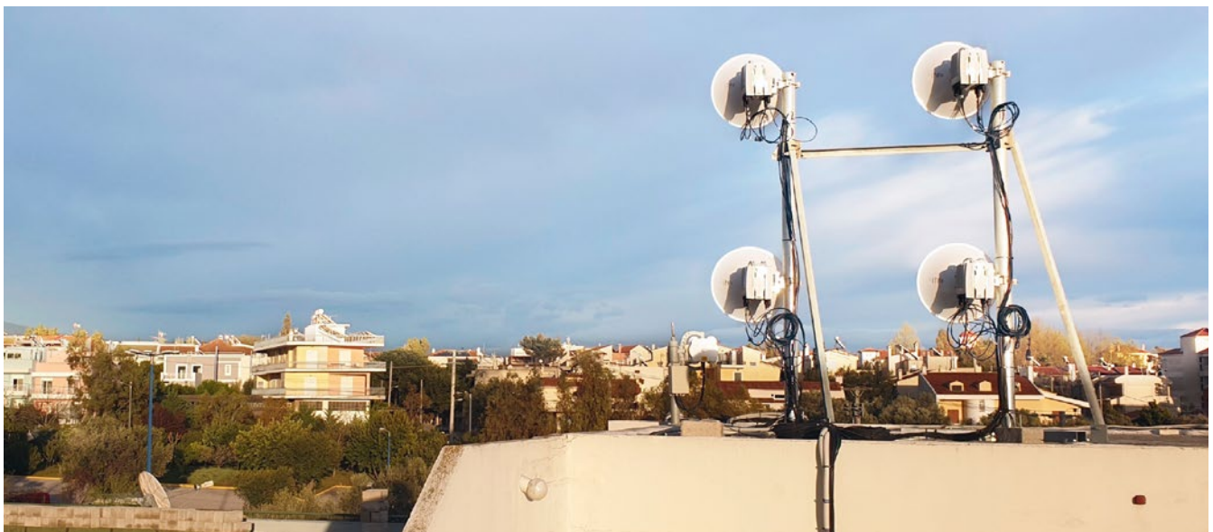
Figure 16: A 100Gbps hop at OTE Academy in Athens, Greece, stretching over 1.5km towards OTE headquarters
