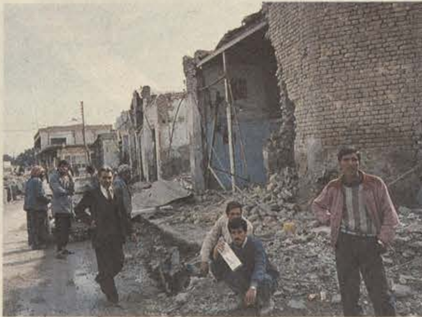
The situation in Kuwait today is very much like that following a disastrous earthquake. Now, it is a matter of rebuilding the country quickly.
