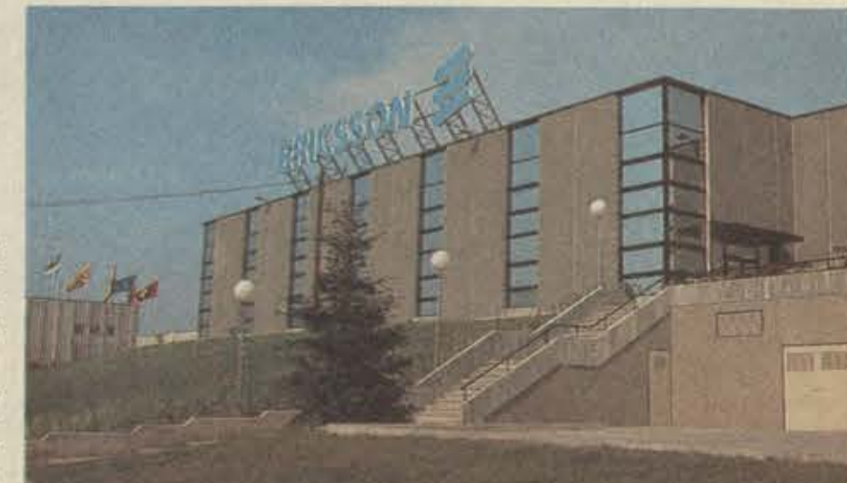
The strict and elegantly designed factory lies in Manresa's new industrial zone, Bufalvent.
