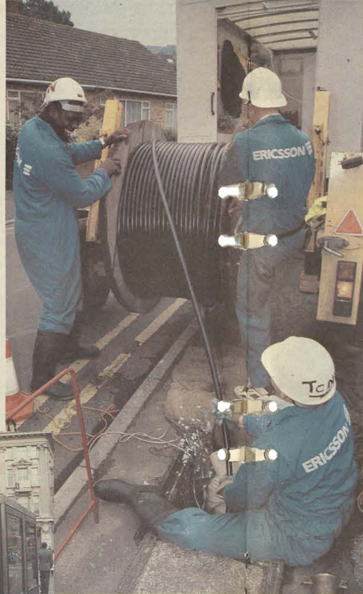
A cable running team in full action in the "cheese metropolis" Cheddar. Here they are laying 530 meters 200 pair cable.
