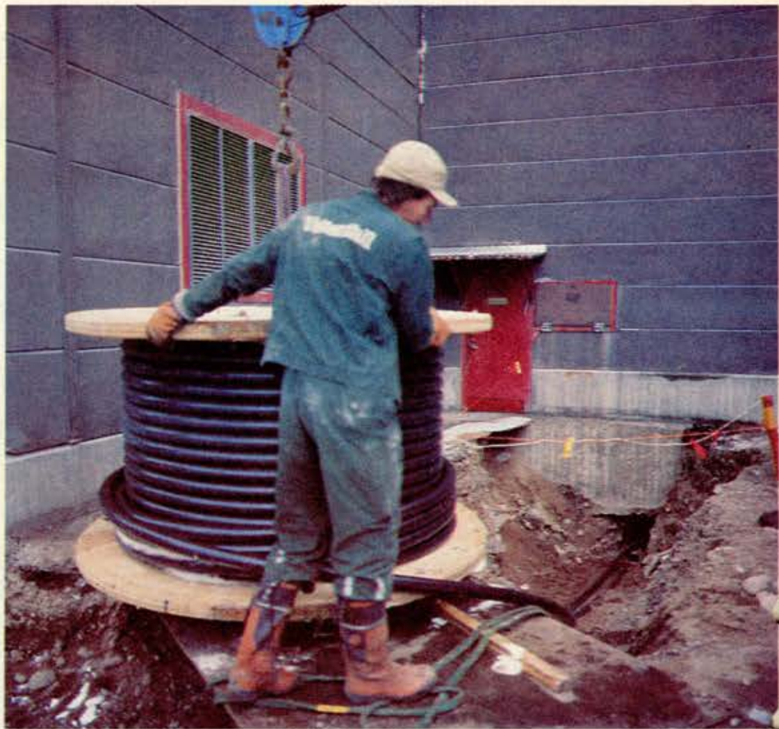
From laying, outside Avesta, of record cable from Falun
