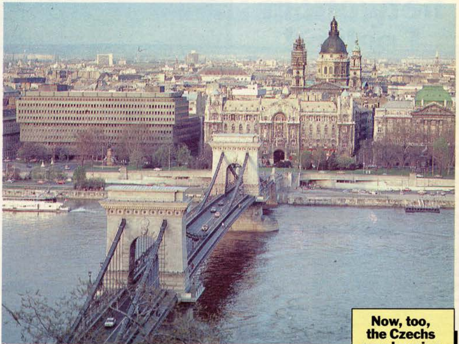
Ericsson has been chosen as a system supplier in Hungary. In 1991 five switches will be delivered to Budapest and the outskirts of the city.
