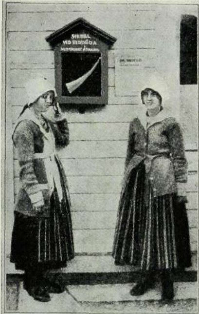
Swedish alarm box. Note horn incased in box. Sender of an alarm in Sweden must have good lungs, instead of trusty fingers.
