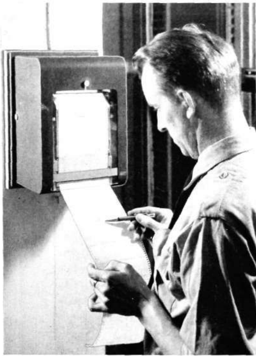
Fig. 7 X 2068 Reading the centralograph fault record in a trunk exchange ARM 20
