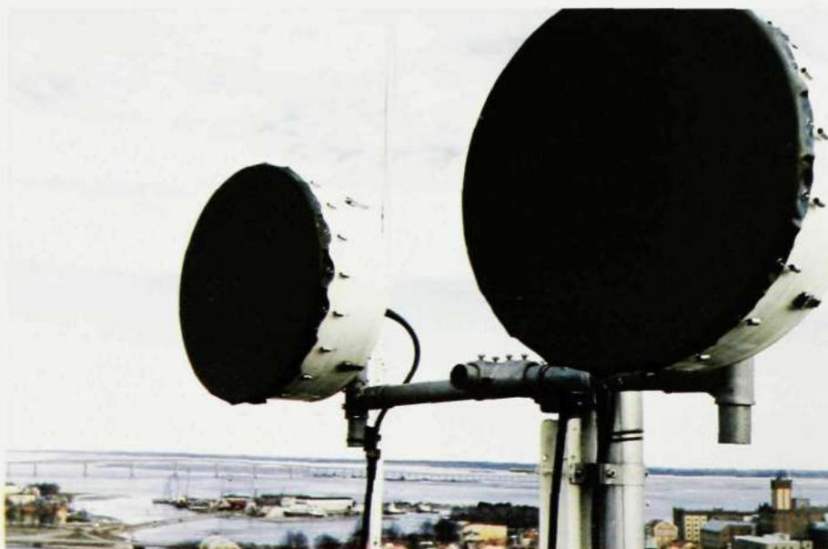
Fig. 11 Two MINI-LINK antennas with radoms installed on the water tower at Kalmar. The antennas are connected to the radio equipment via short elliptical waveguides
