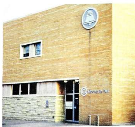
Fig. 4 The Mountain Bell exchange building in Cañon City
