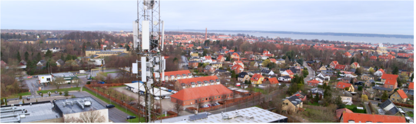
A "drone's eye view" of a network tower site
