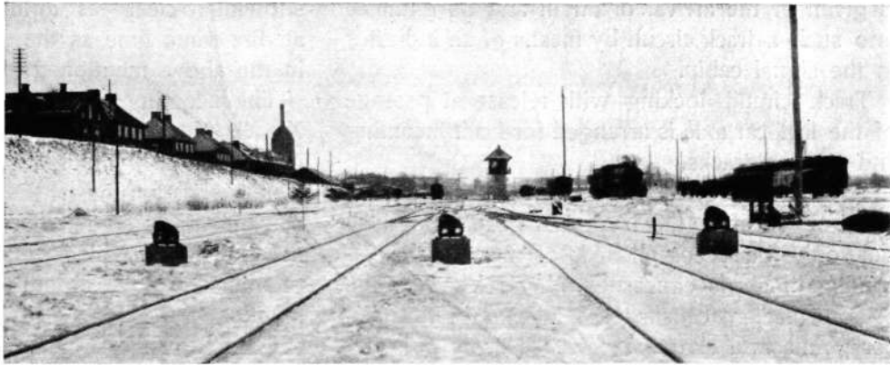
Shunting Signals M I —M III , Arranged as Dwarf Signals.
