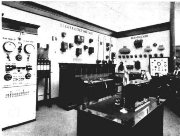
R 3 Electric meters and fire-alarm apparatus.
