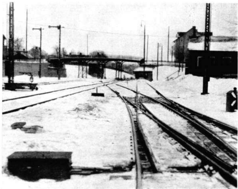
R 42 Double Point and Starting Signals at South End of Station Yard.
