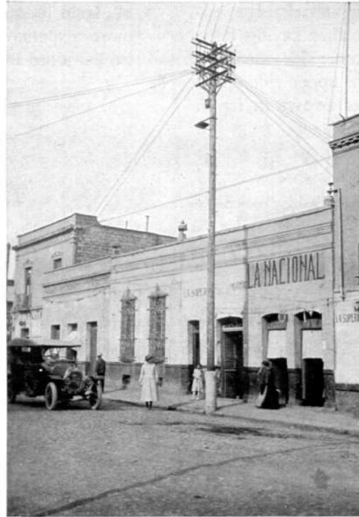
R 176 Fig. 10. 40-foot Distribution Pole with Pole Support. Mexico D. F.
