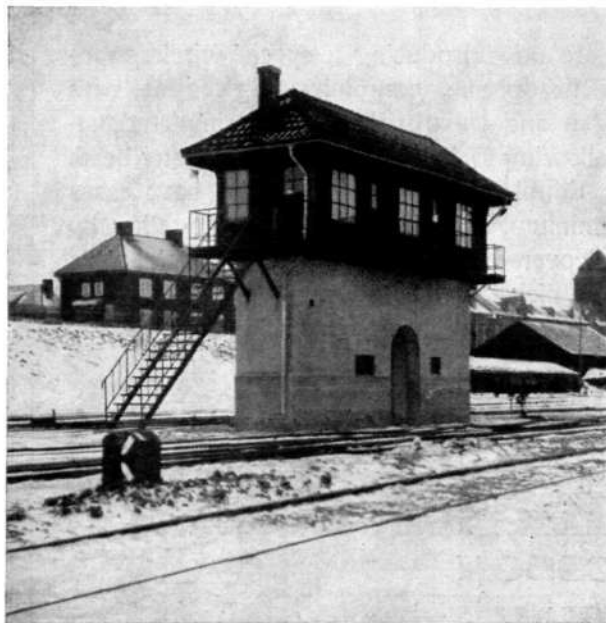
R 40 Signal Tower at North End of Station Yard.
