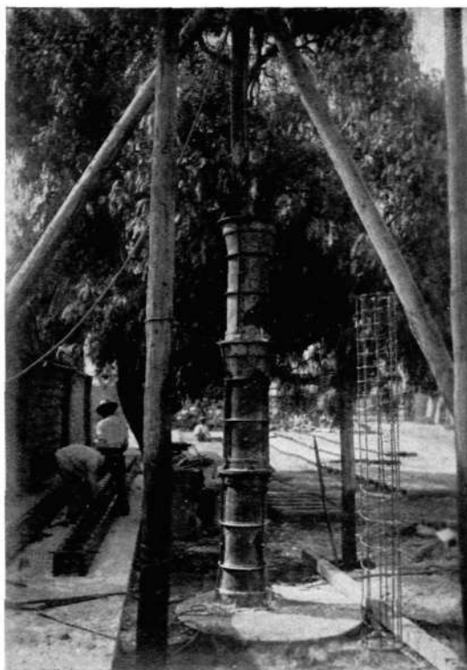
R 174 Fig. 8. Form and Reinforcement for Pole-Support.
