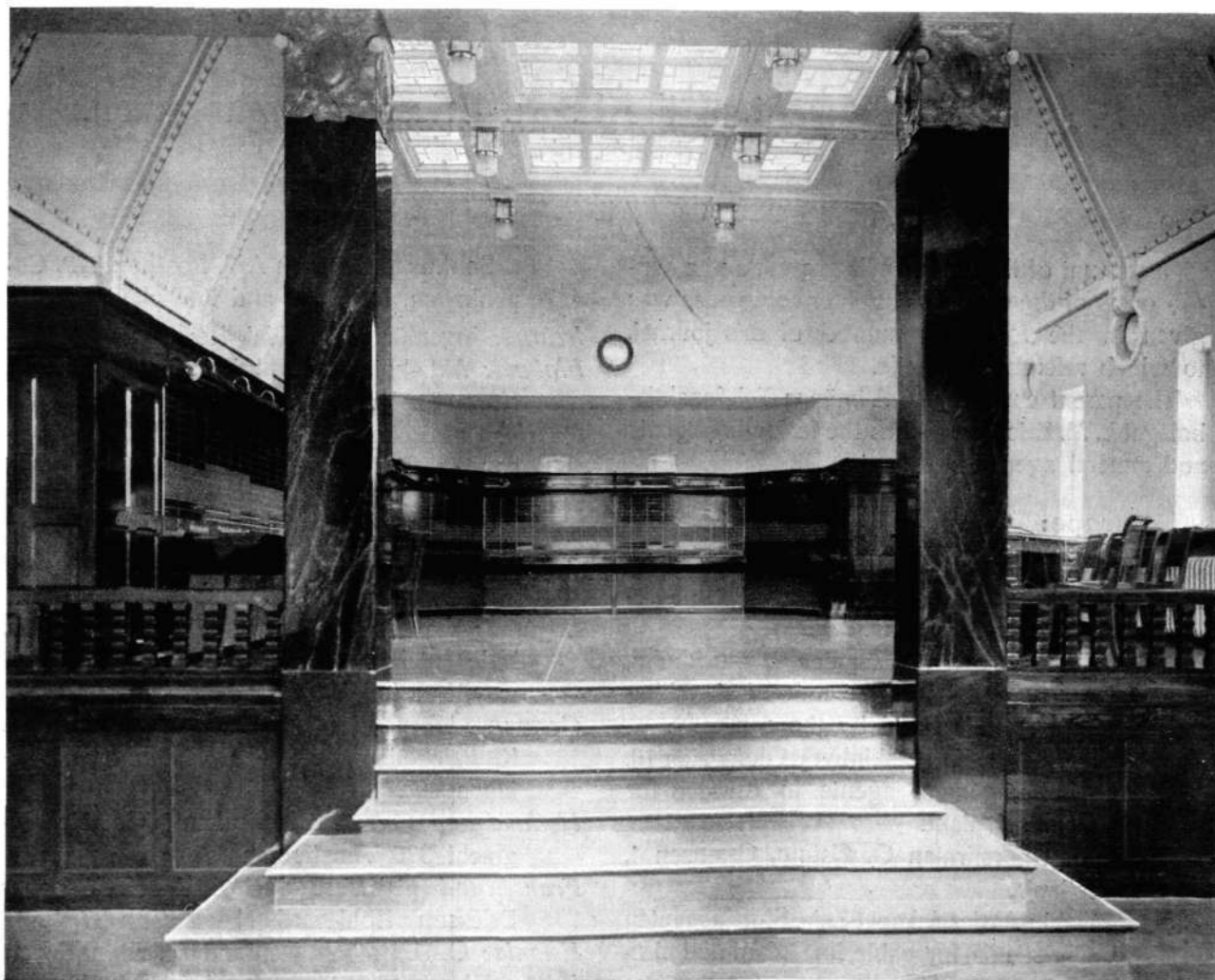
OPERATING ROOM OF THE NEW ÅBO TELEPHONE EXCHANGE
