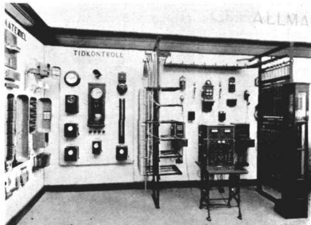
R 4 Time control system and line equipment.
