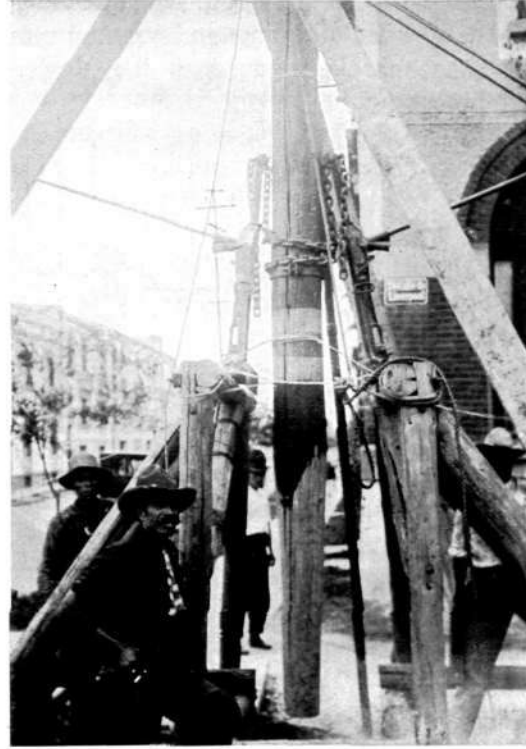
R 173 Fig. 6. Setting of Amputated Pole in Pole-Support without Interrupting Service.
