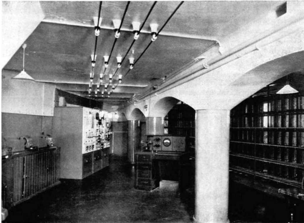
Fig. 3. Main Distributing Frame and Power Board.
