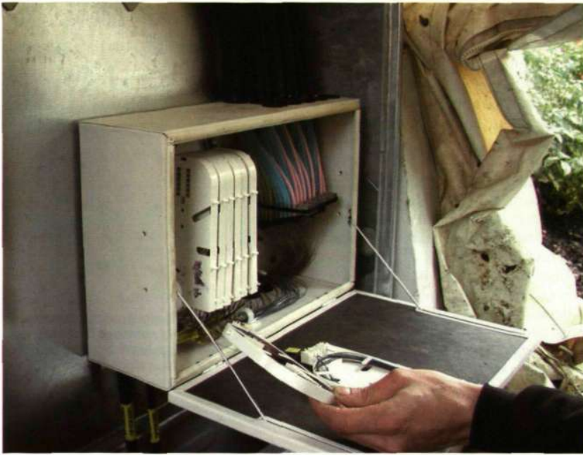
Figure 7 Ribbonnet duct-/fiber-jointing cabinet for outdoor use, for example, in residential areas.
