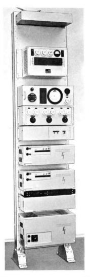
Fig. 9 X 2319 Power Supply Bay for an auxiliary repeater station
