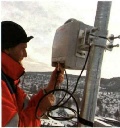
Figure 8 Installing MINI-LINK.
