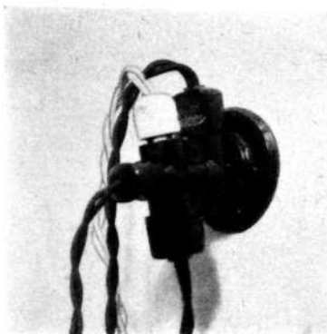
Fig. 4 »Multiple wall socket» a dangerous makeshift when there are not enough wall sockets
