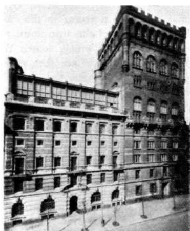
Fig. 1 Zielna telephone exchange at Warsaw
