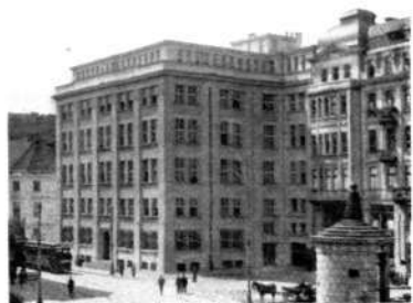
Fig. 2 Tłomackie automatic exchange
