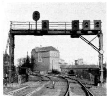
Fig. 5 Signal-bridge with signals for traffic with harbour
