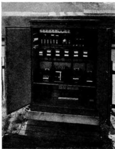
Fig. 5 Relay cubicle
