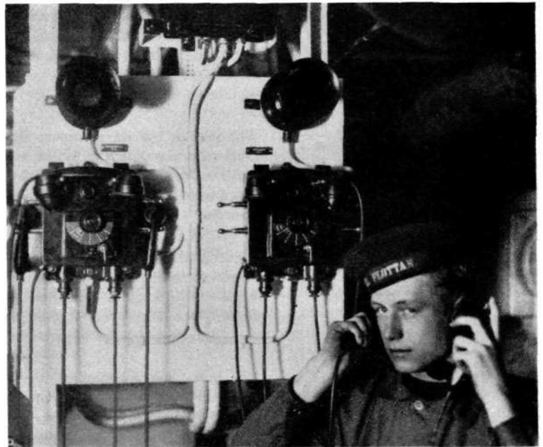
Fig. 7 Wall instruments with signal horns
