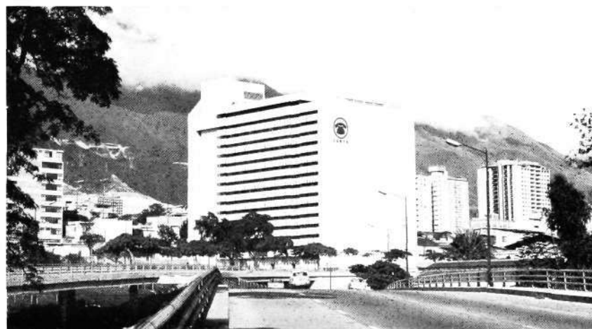
The first stage of the new Venezuelan telecommunications centre, CENTRO NACIONAL DE TELECOMUNICACIONES, was officially opened on December 15, 1967, by President Leoni. The photograph shows the main building of CANTV on Avda. Libertador, Caracas.
