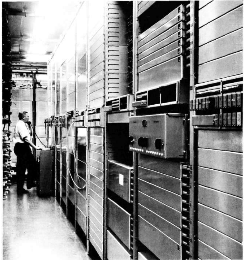
Fig. 2 Intercontinental transit exchange, L M Ericsson type ARM 201, in Montreal
