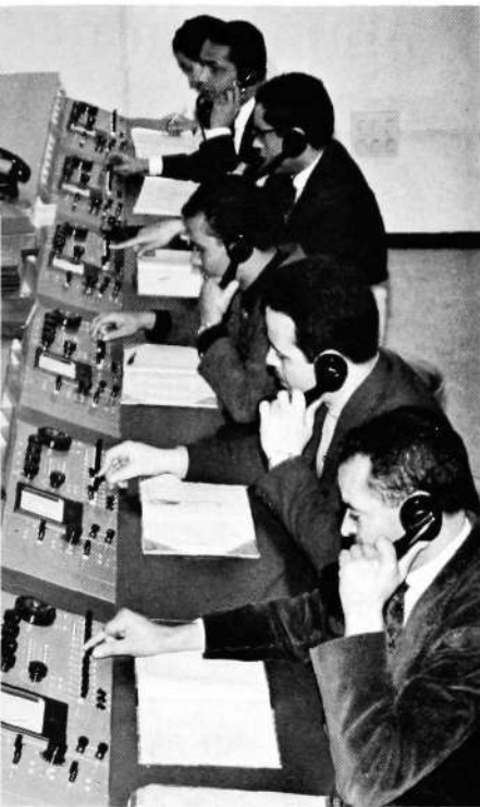
Fig. 3 Test desk for testing subscriber's lines and receiving complaints
