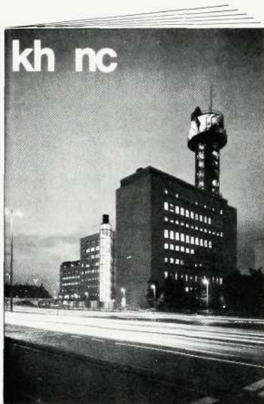
The telephone building in Copenhagen is the illustration on the cover of a booklet on a new computer-controlled exchange, kh nc.
