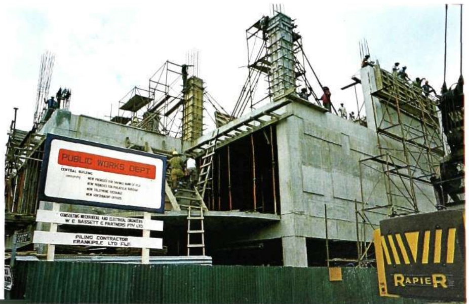
Fig. 1 Building a telephone exchange in the town of Suva
