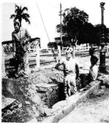
Fig. 2 Locating a cable to avoid injury during street excavation
