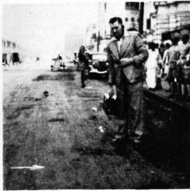
Fig. 1 Locating a cable bend
