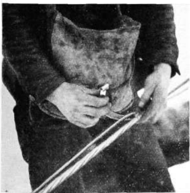
Fig. 8 Mounting of cable suspenders
