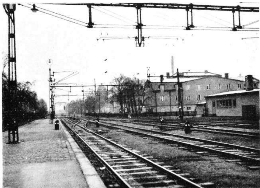
Fig. 1 Dwarf signals in the station track area
