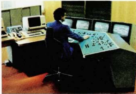
Fig. 15 A control position with four colour video displays and one black and white display for information in the form of text
