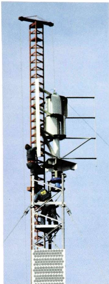
Fig. 16 Mounting of the wind turbine
