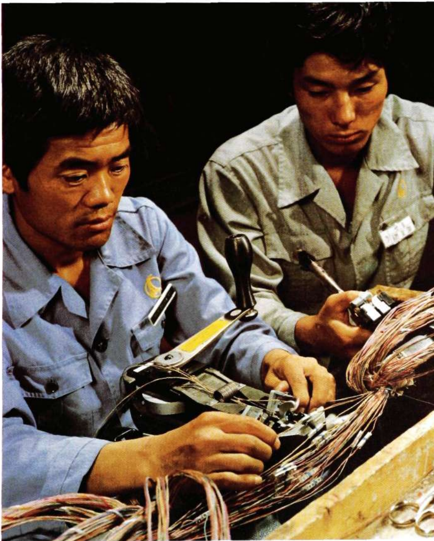
Fig. 13 Practicing cable jointing at the Dong Ah training centre
