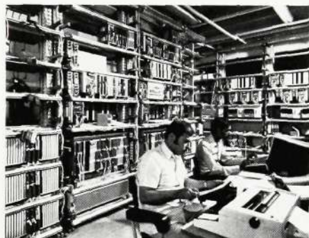
COVER Installation testing of an AXE 10 exchange in Saudi Arabia
