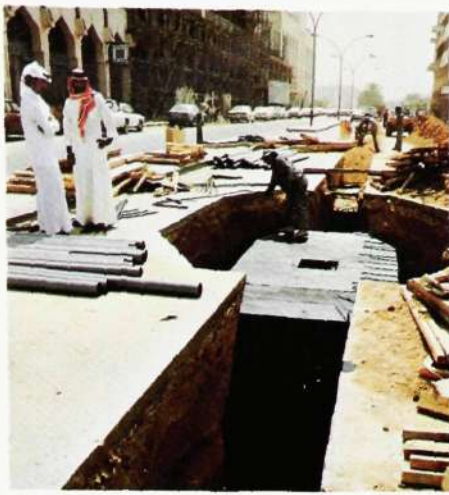
Fig. 3 Installation of ducts for the subscriber network in Riyadh
