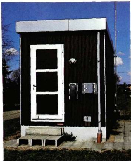
Fig. 7 Cabin in the station area containing the equipment for one track sector
