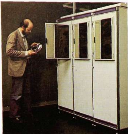
Fig. 7 Magnetic tape units for charging and statistics
