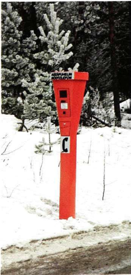
Fig. 1 The shape, colour and reflecting labels of the emergency telephone column makes it clearly visible
