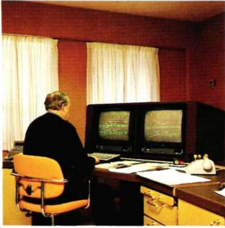
Fig. 15 The control office for Malmö railway yard area
