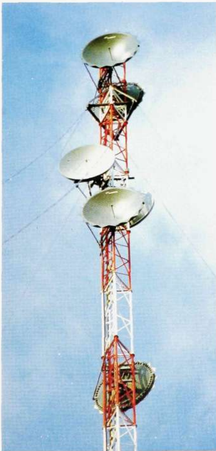
Fig. 3 The building and mast of a radio relay link station in Ruukki
