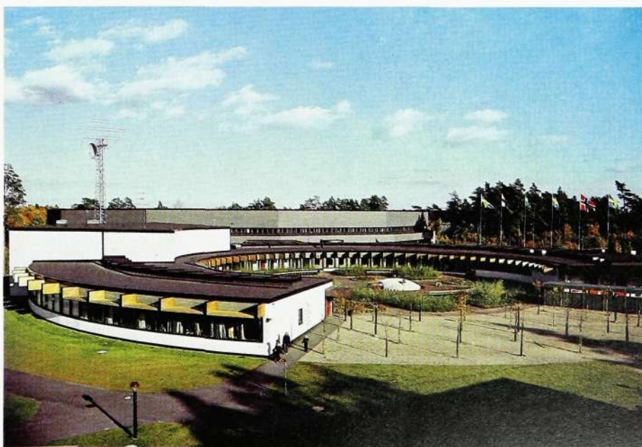
Fig. 11 The Telecommunications Training Centre at Kalmar, in south-east Sweden
