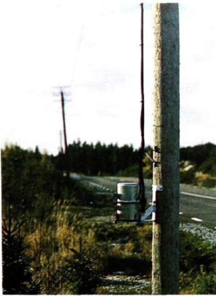
Fig. 3 A pole with a housing for connecting a screened TUKA cable
