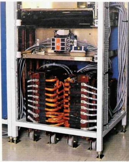
Fig. 8 The transformers are equipped with wheels, which simplifies their handling during installation. The front cross-member of the rack is removed when the transformers are installed. Clear labelling ensures correct connection to the secondary side. The fixed cables on the primary side are connected direct to the mains contactor
