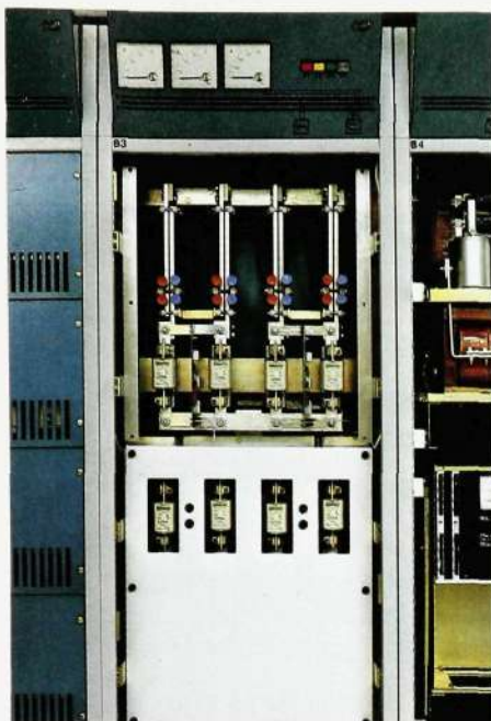
Fig. 11 Low-ohmic distribution Cartridge fuses for a maximum of 400 A
