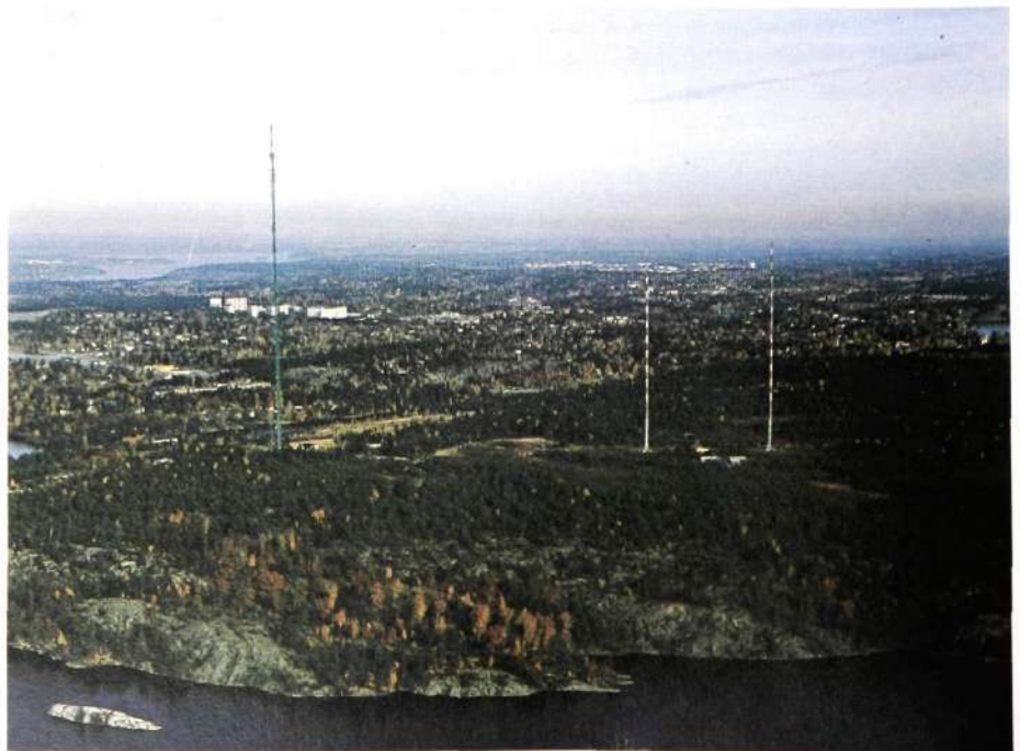
Fig. 1 The base station for mobile telephony at Nacka, outside Stockholm, Sweden. As far as possible, existing radio and TV masts and buildings are used for the base stations. In this case the mobile telephone antennas are placed in the left-hand mast, at a height of approximately 200 m. The other base station equipment is placed in the building immediately to the right of the mast.
