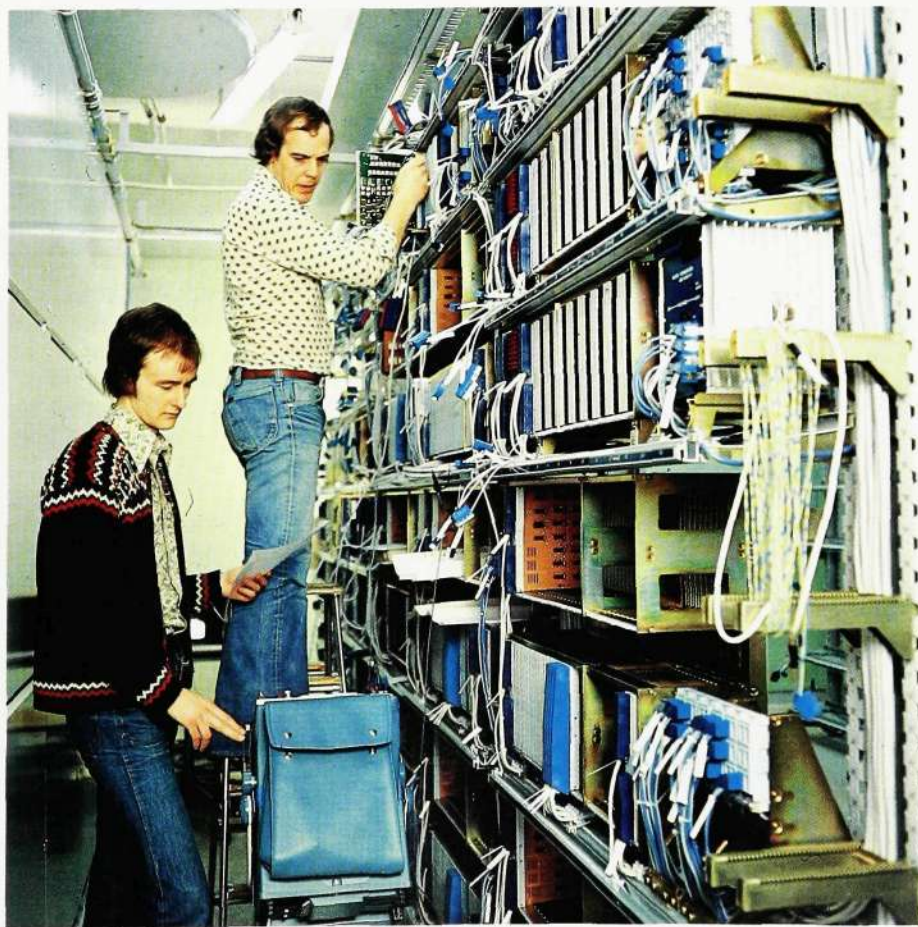
Fig. 5. The Södertälje exchange during the installation
