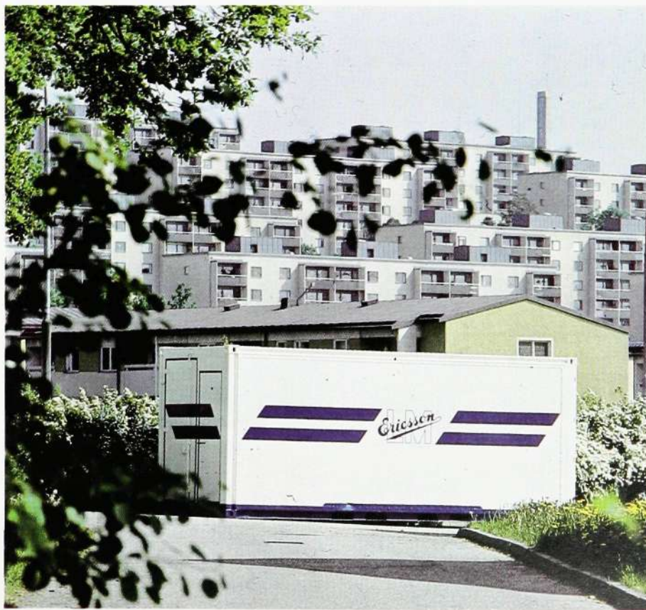
Fig. 2 Digital subscriber stage placed in a container for remote location
