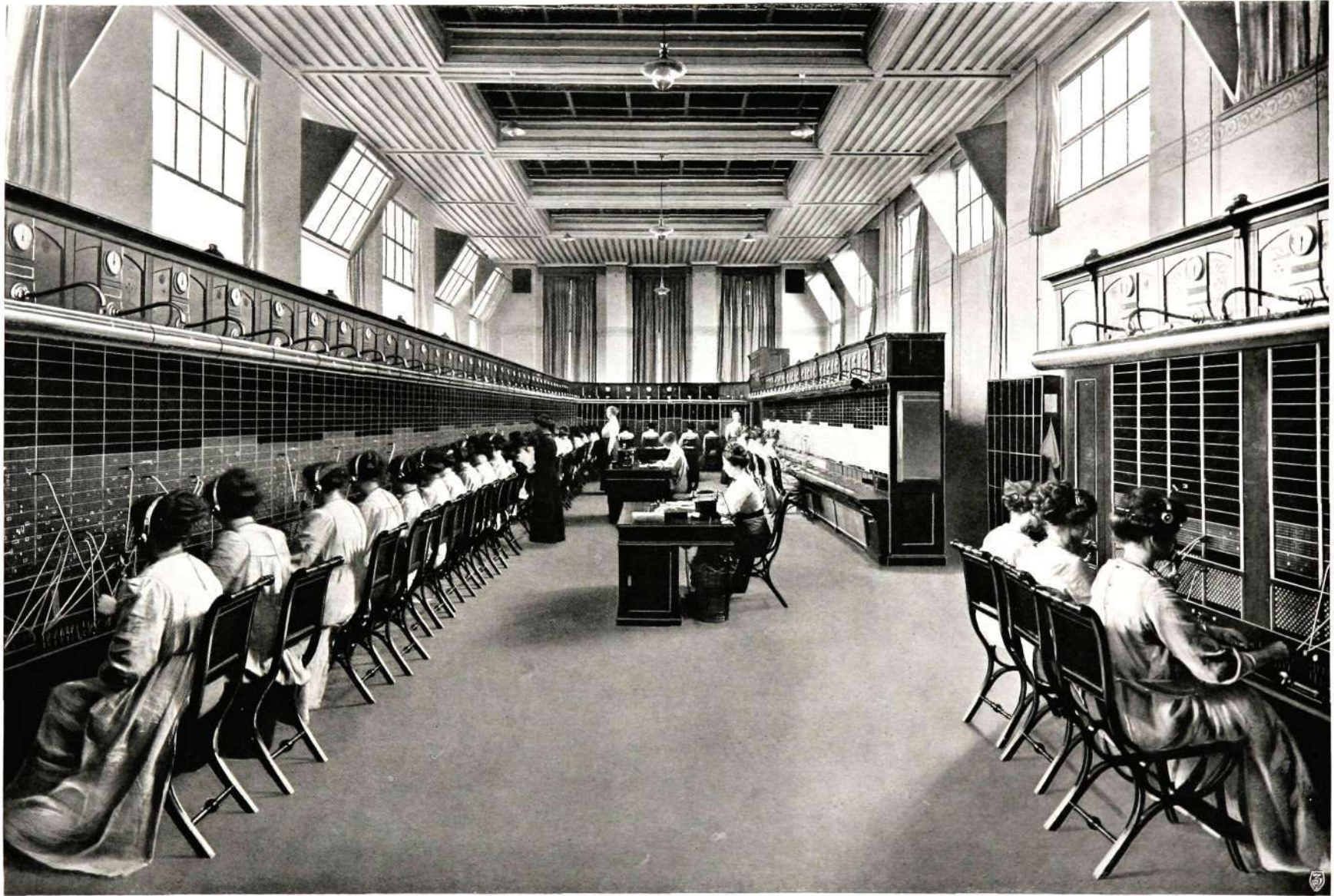
The Telephone Exchange at the Hague, Holland Local Positions
