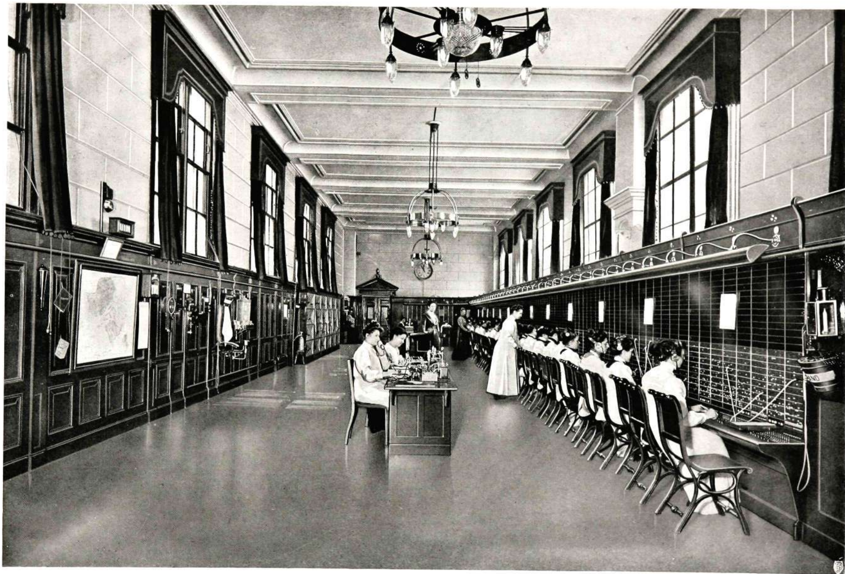
The Rotterdam Telephone Exchange, Holland Local Positions
