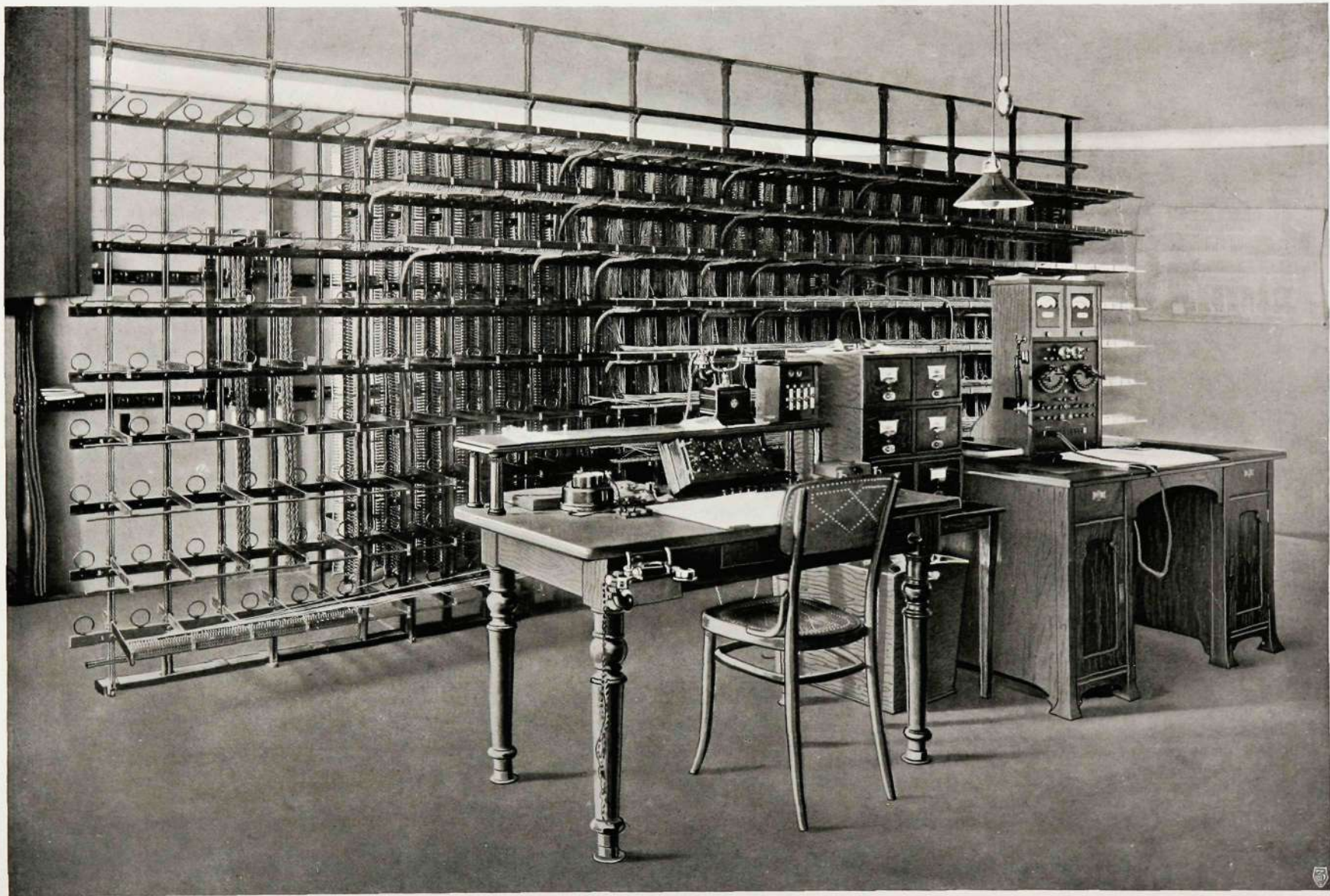
The Helsingborg Telephone Exchange, Sweden Cross Connecting Frames
