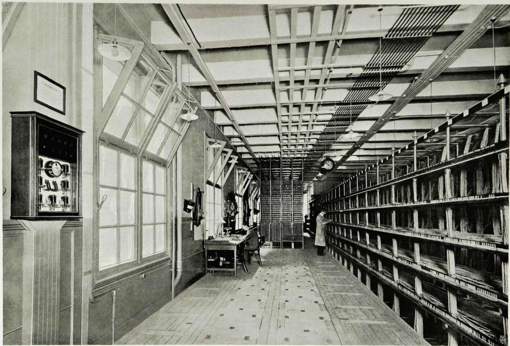
The Rotterdam Telephone Exchange, Holland Cross Connecting Frames
