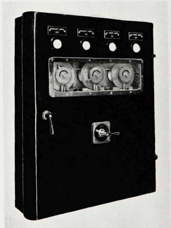
Fig. 5—"Actadis" Mechanical Time Switch Cabinet
