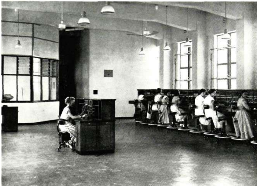
Fig. 7—The Manual Switchroom, Mombasa
