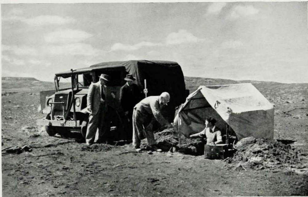
Fig. 6—Laying the Cable
