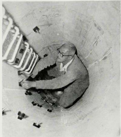
Fig. 3—Inside the Pylon
