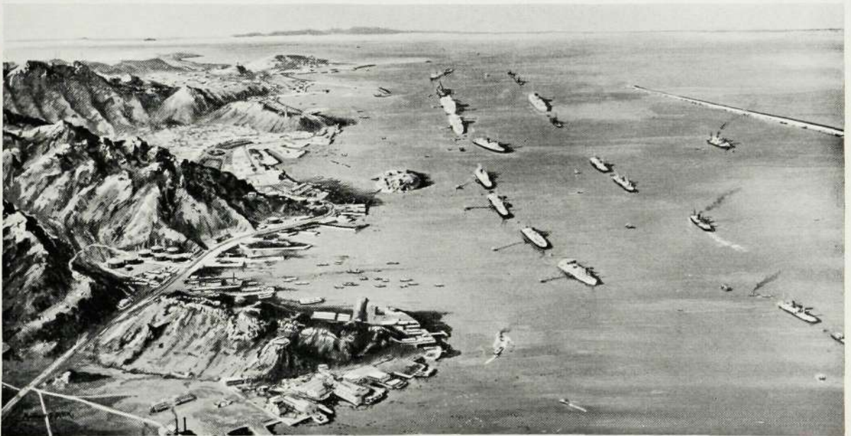
Fig. 1—Bunkering Facilities at Aden. Little Aden is on the horizon
