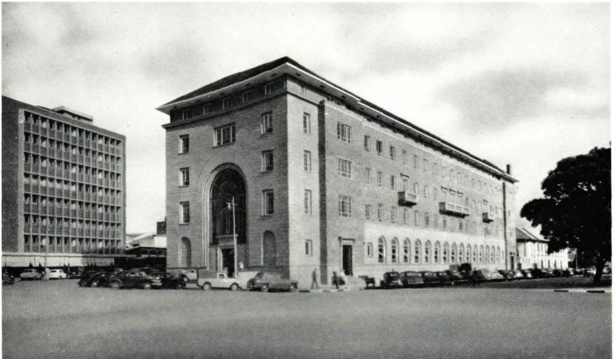
Figure 1—Salisbury Central P.O. accommodating one of the Telex exchanges
