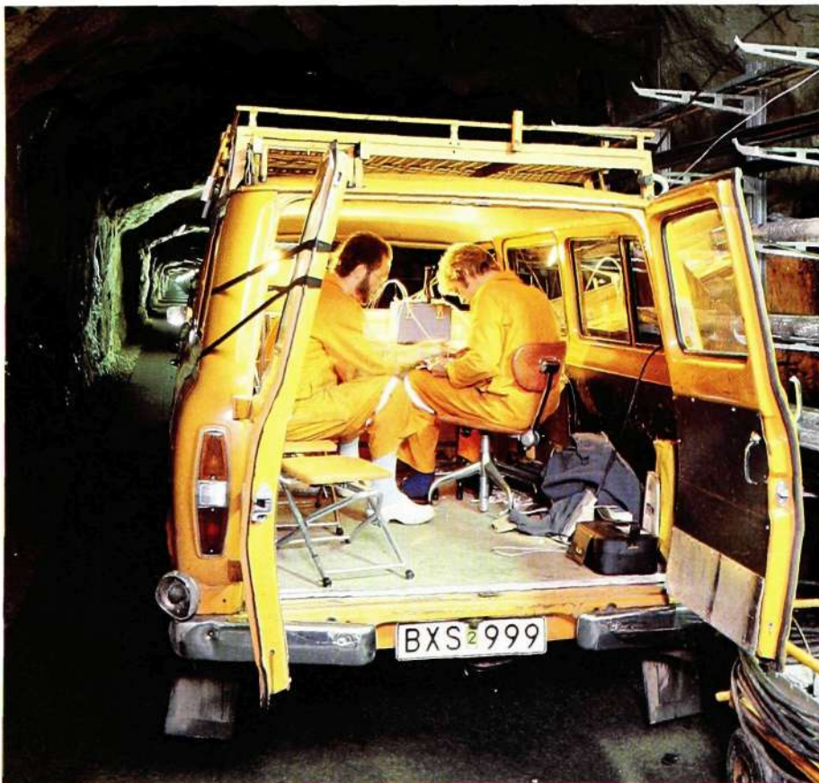
Fig. 5 Joining work station for fibre cable set up in a van
