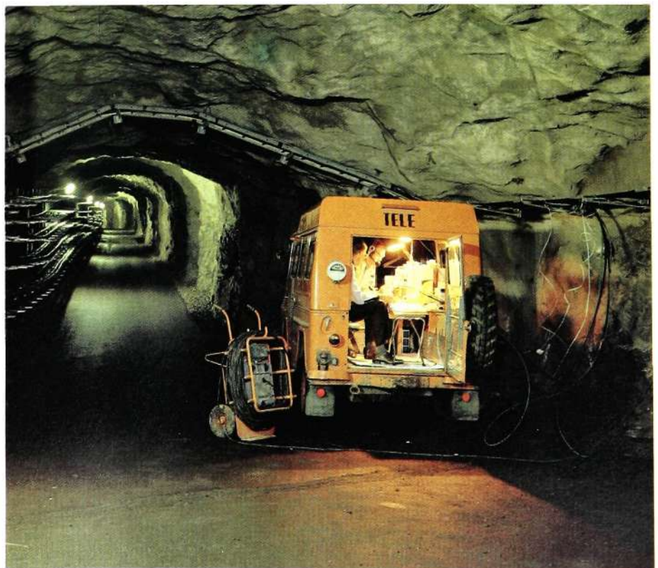
Fig. 1 The tunnel in Stockholm where the field trial FOK-79 was carried out
