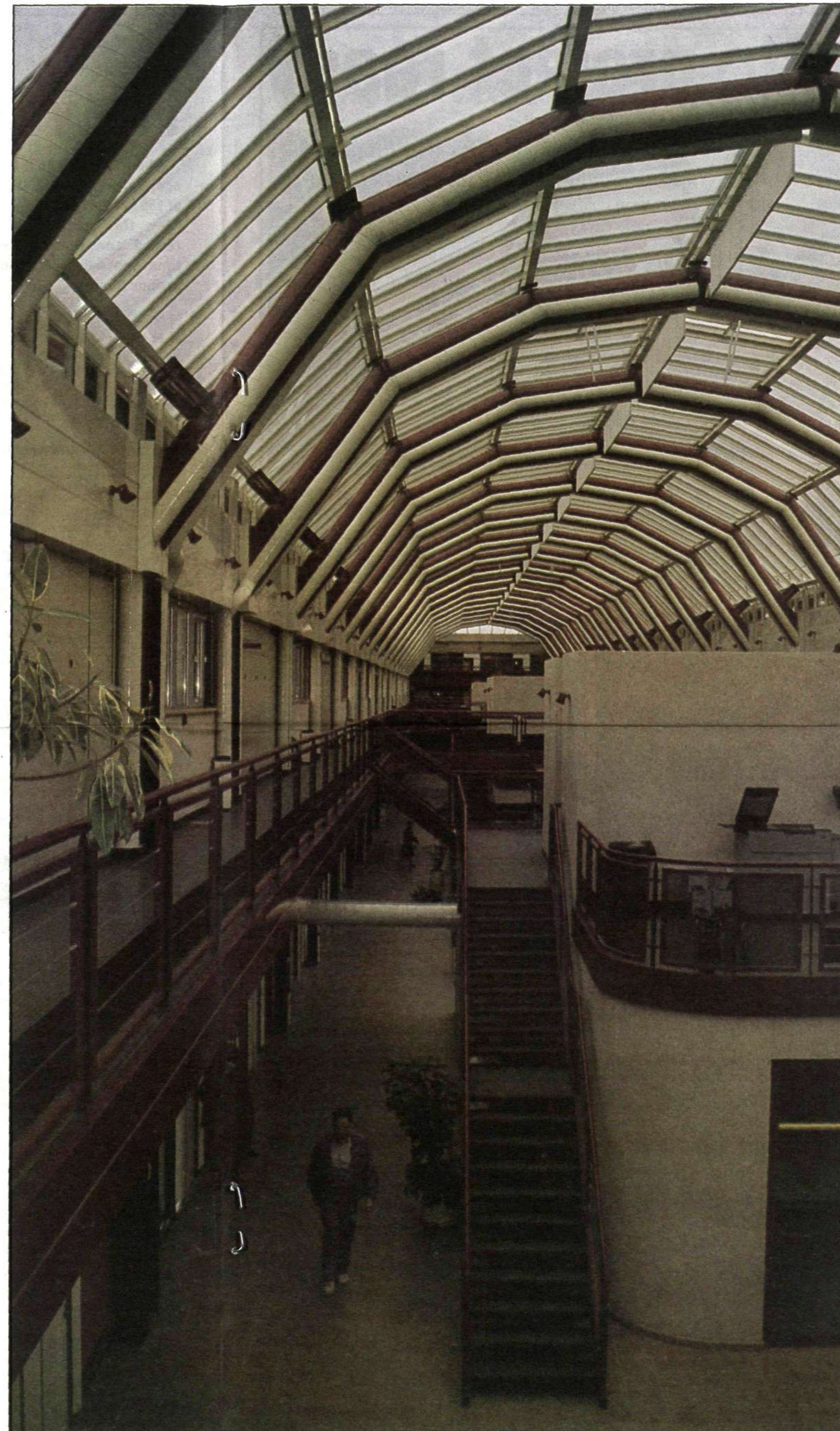
The office, with the administration side, construction and development, and installation testing is in Massy, a Paris suburb. A modernized older factory site, with lots of space and greenery, houses the new "French" AXE culture.
