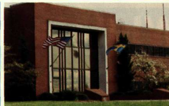
Ericsson/GE plant in the U.S. is located in Lynchburg, Virginia, on the East Coast. Some 2,000 people work there with design, production and supply of terminals and systems within mobile communications.
