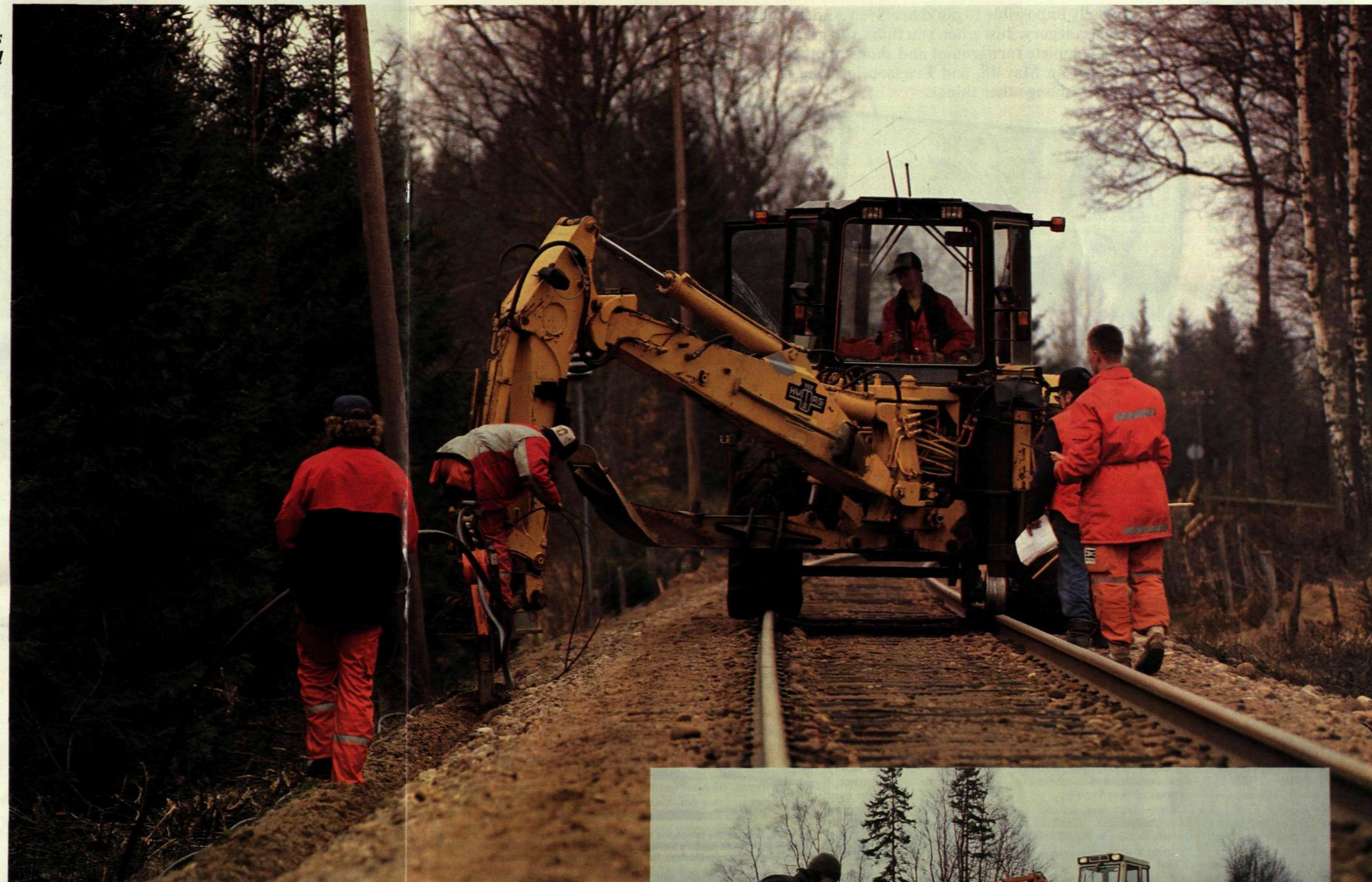
Plowing for laying of optocable along tracks in the Värnamo-Halmstad strip.
