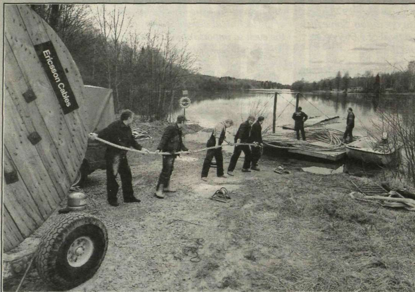
Laying underwater cable. Photo: Thord Andersson
