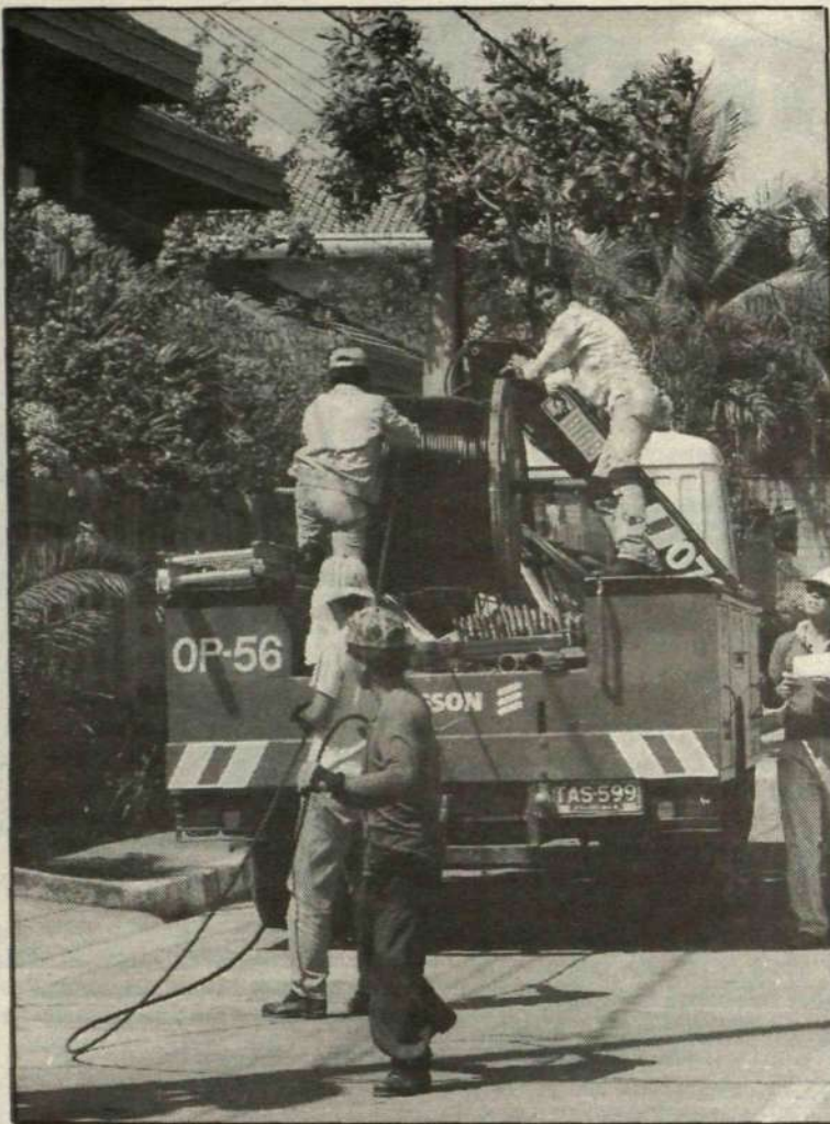
Philnet Ericsson previously carried out several network construction projects in Manila.
