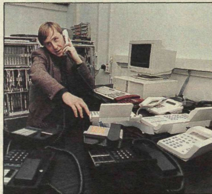
One of the major challenges for the company is to help customers to build up their own internal network. An important part of this work is to test modems and other associated equipment.
