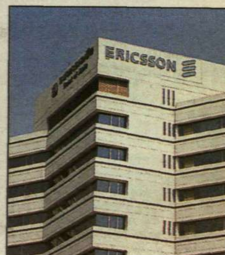
Ericsson's Bangkok office is located near the Don Muang Airport.
