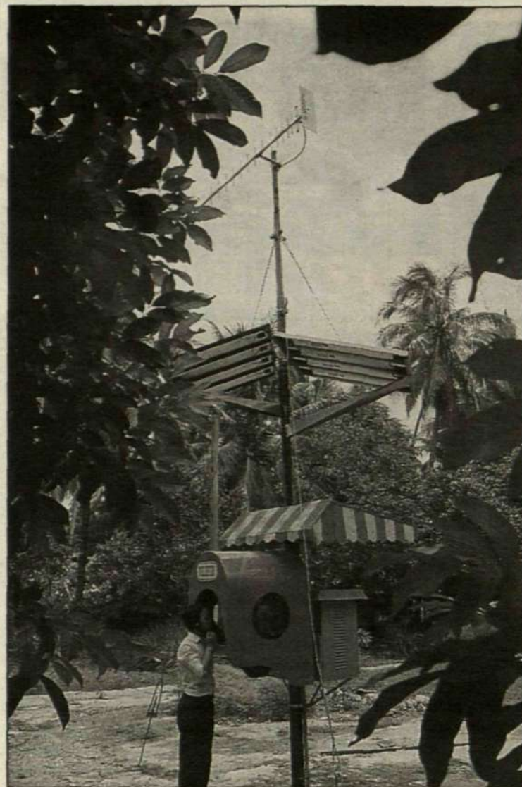
Ericsson has delivered radio technology to Malaysia for many years. Remote telephone "kiosks" that are connected to the fixed network with radio links are an unusual feature of the Malaysian system.
