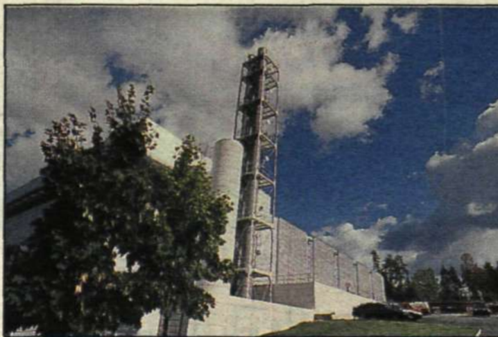
On 120 pillars bolted fast in the rock foundation, Ericsson's new microtechnology plant rises toward the sky. The firm footing makes the building vibration-free.
