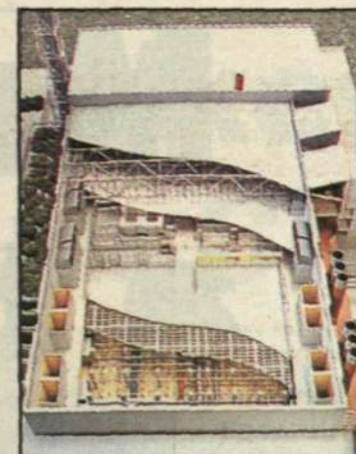
A model in the visitor's gallery shows the plant's construction, with pillars, a waffle-like floor, clean rooms, air shafts, the filter ceiling with specially designed rafters and the various level.
