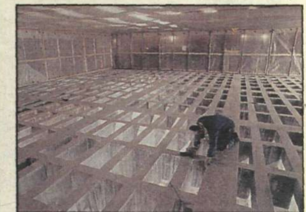
The support level with the supporting pillars for the grated floor on the clean rooms. This level contains the distribution system for resin, air, electricity, gases and chemicals. The floor of the support level is separated from the pillars and walls and rests on a one-meter layer of special gravel that absorbs vibration from the bedrock.
