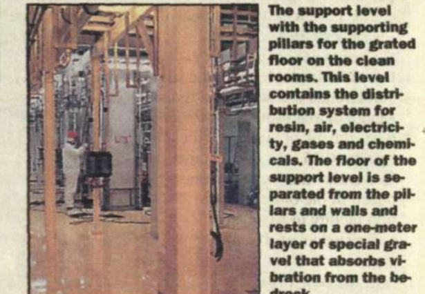
The entire plant is a demonstration of high technology, with an integrated clean room and advanced systems for air, water, gases and acids, as well as the very latest production equipment in the industry. Cleanliness and freedom from vibration are the two most important parameters for advanced semiconductor manufacturing.
