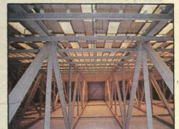
The plant's ventilation system circulates 1.3 million cubic meters of air each hour. This means that the air in the plant is changed 400 times per hour.
