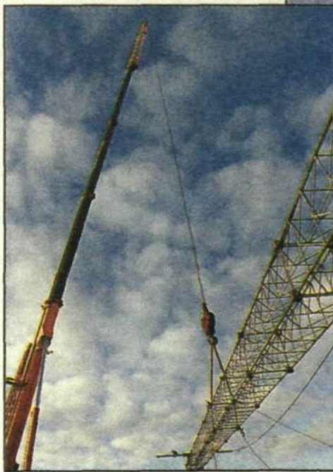
Going up! Despite the mast being 51 meters high, it weighs only approximately 1,500 kg.
