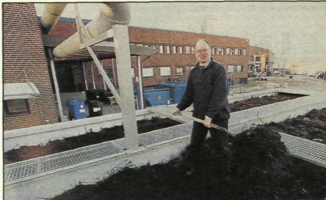
The man behind the biological purification process, Ulf Ljungberg, is seen in the center of action. In this biological filter comprising soil, peat and heather, solvents are transformed into the harmless substances of water and carbon dioxide.
