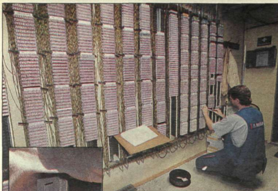
Above: Telia installed more than 200 kilometers of cable in the Ullevi Stadium area alone for World Championship traffic. Telia installer Toni Spets is shown working at one of the temporary cross-coupling modules.
