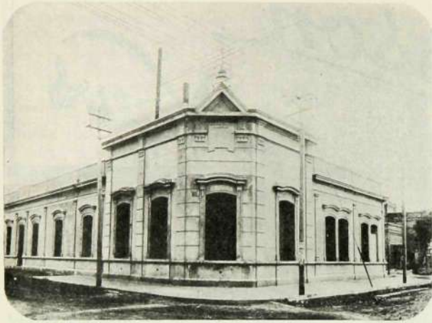
R 822 The Resistencia Exchange Building.
