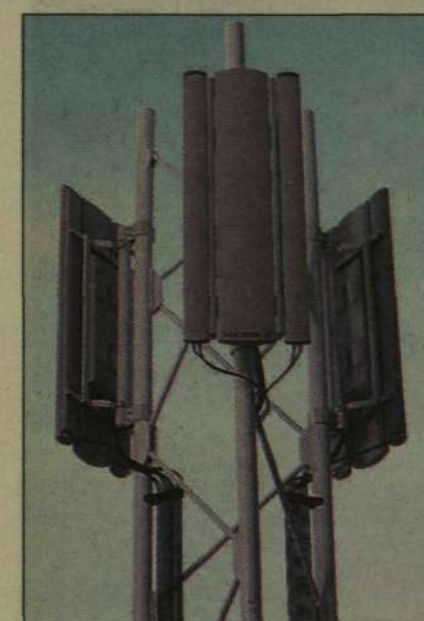
In "active antennas," part of the base station is moved up into the antenna to provide greater coverage ranges.
