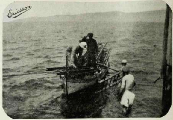
R 1043 Transport of cable ladder.
