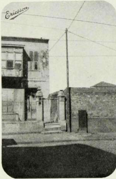
R 1042 Pole with box.
