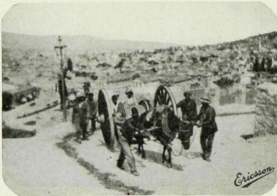
R 1044 Transport of cables.
