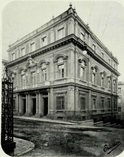
R 1071 Fig. 4. Exterior of the «Amedeo» Telephone Exchange.
