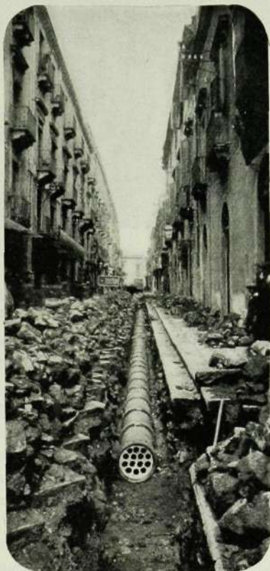
R 1143 Cable-laying in Catania.
